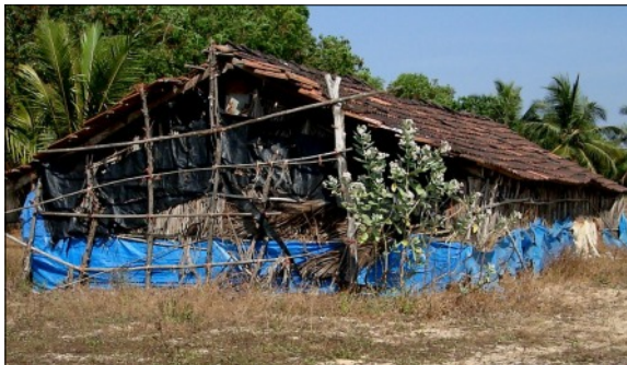
Figure 20. et-houses are key to the longevity of sewn fishing craft: a) laterite piers and tiled roof at Benaulim; b) mixed construction in the dunes at Fish Road; c) small pirogues under palm-thatch and timber at Nuem. Author.
